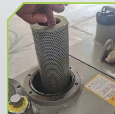
Fuel tank filter maintenance 工作油箱滤芯更换
