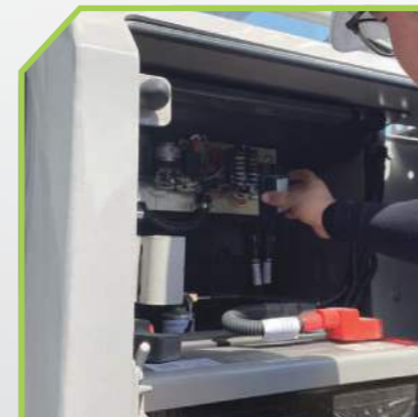
Replacing fuse 保险更换
