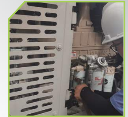
Fuel filter maintenance 燃油滤更换
