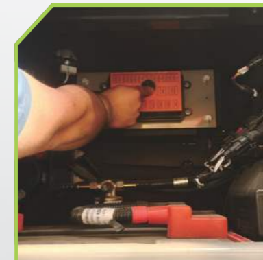
Replacing fuse 保险更换
