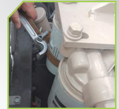
Fuel filter maintenance 燃油滤更换
