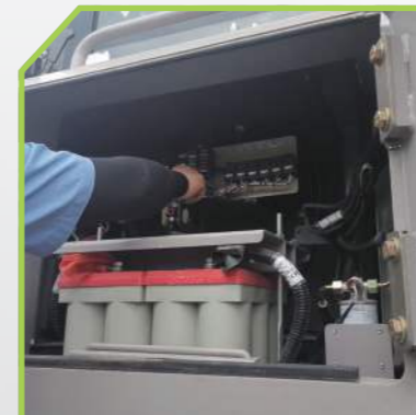
Replacing fuse 保险更换
